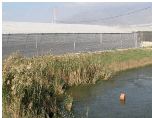
Figura 26. Reservoir that collects rainwater falling on greenhouses
